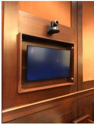
2. New digital control system - New AMX NetLinx digital control system with AMX touch panels for the Judge, Deputy and Evidence cart. AMX control systems are required maintain consistency and compatibility with our other courtroom control systems. AV source switching system through control panels located at the judge, deputy, and evidence cart locations. The control interface must look and function the same as the control system as specified by the Court.
